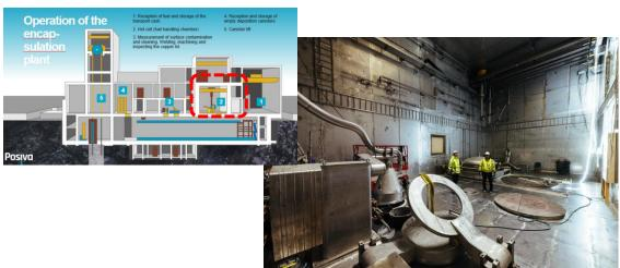
Docking stations for the canister and the fuel transport cask, drying station for spent fuel at the fuel handling cell
